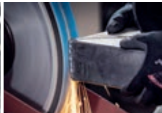
Levelling of welded seams
